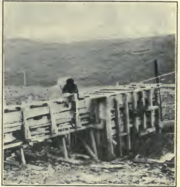
PENSTOCK AT MIOCENE DITCH SUPPLYING ELEVATOR.
